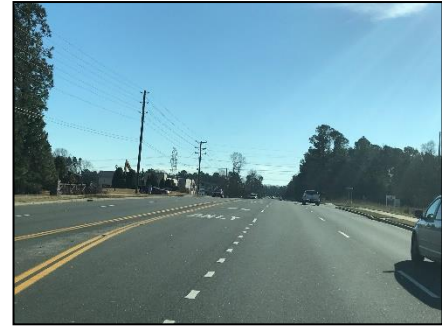
Example of a principal arterial: SC 160
